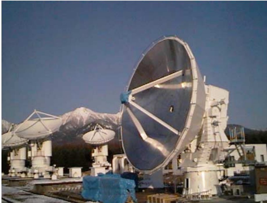
Figure 1: A new 10 m submillimeter telescope was installed at Nobeyama in February 2000. The other telescopes on the background are elements of the Nobeyama Millimeter Array. The size of the receiver cabin is 3.2 x 2.2 x 1.8 m 3 including an annex.
